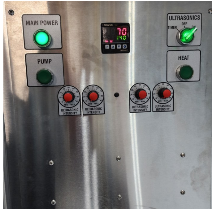
Figure 11 Generator Manual Control On
