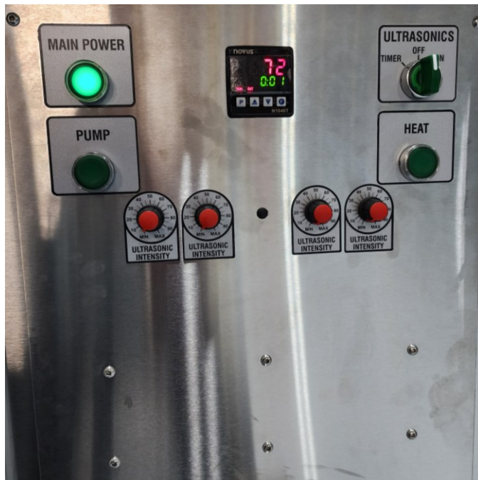
Figure 10 Generators Manual Control Off
